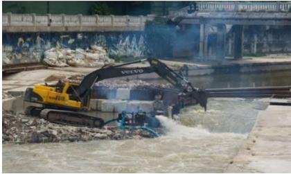
Fig 3 Workers dredge garbage and silt from a storm drain near the Pasar Seni LRT Station following flash floods in March 2017
